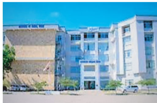
One of the ultra-modern buildings of ISW at Kijitonyama in Dar es Salaam
