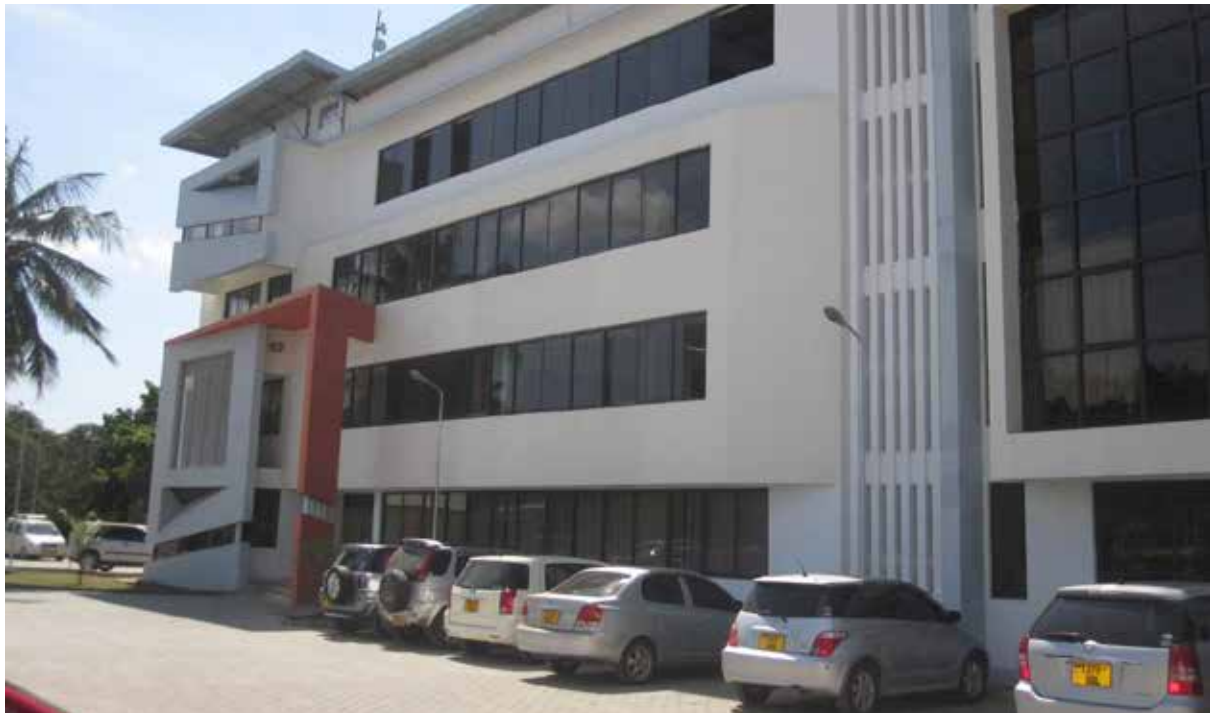
New building for staff offices and students' classrooms at DUCE
